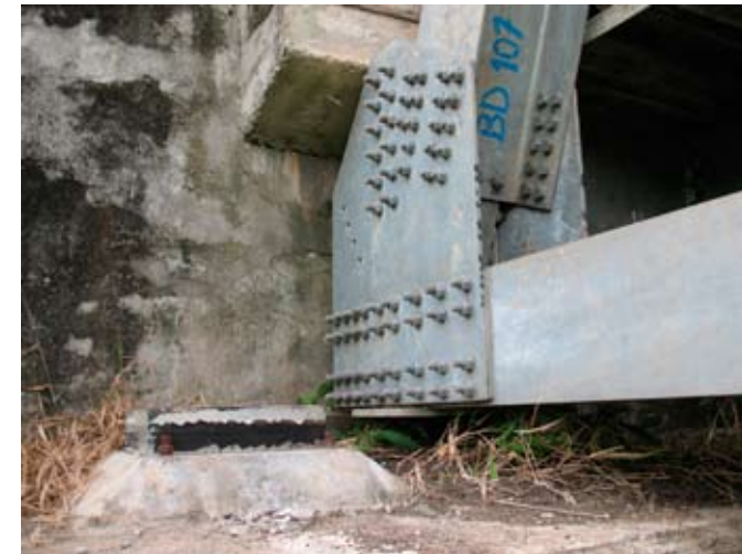
Figure 17. This photograph shows a steel truss bridge located in the earthquake-impacted area. Note that the superstructure did not sustain any damage. However, the bridge had an inadequate transverse shear key, and its abutment bearings had insufficient movement capacity. The steel members in this bridge appeared to be undamaged.
