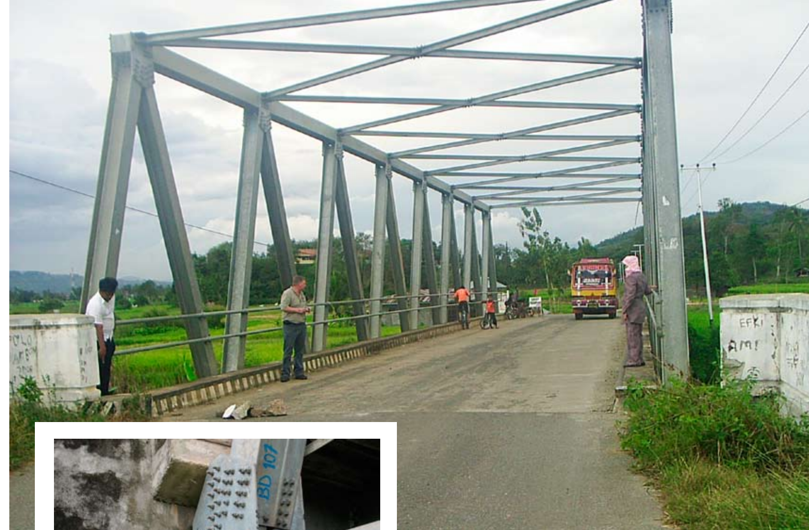
Figure 17. This photograph shows a steel truss bridge located in the earthquake-impacted area. Note that the superstructure did not sustain any damage. However, the bridge had an inadequate transverse shear key, and its abutment bearings had insufficient movement capacity. The steel members in this bridge appeared to be undamaged.
