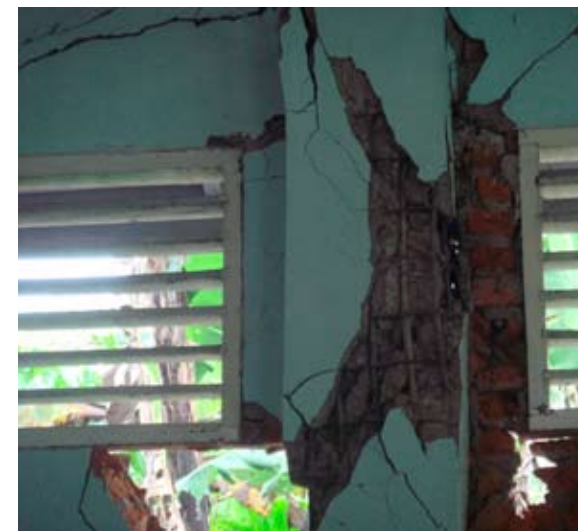
Figure 8. These photographs show out-of-plane failure of URM walls. These URM buildings do not have adequate floor diaphragms, and URM walls are not positively connected to the perimeter bond beams and columns. As such, they are not restrained against out-of-plane failure.
