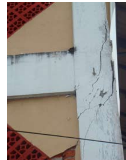
Figure 9. The beam-to-column joints for the concrete moment frames do not use ductile detailing. The reinforcement steel does not extend sufficiently into the joint, nor does it have adequate development length. Furthermore, the joints are not confined and hence are susceptible to shear failure.
