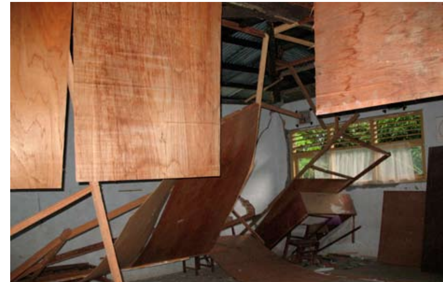
Figure 15. The photographs show nonstructural damage to a school building. This building did not sustain any structural damage. However, the ceiling and soffit collapsed. Unless these elements are properly designed and anchored, they are life-safety hazards. For this school building, ceiling panels collapsed in the classrooms, and roof soffit panels dislodged.
