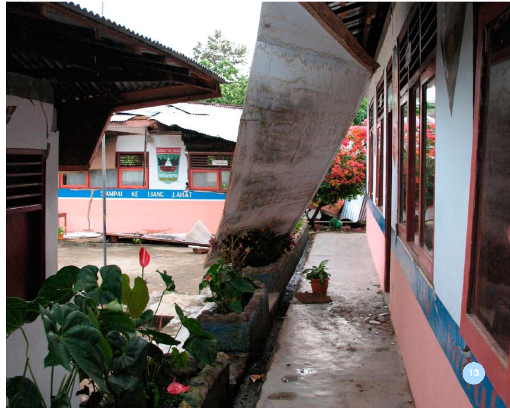
Figure 15. The photographs show nonstructural damage to a school building. This building did not sustain any structural damage. However, the ceiling and soffit collapsed. Unless these elements are properly designed and anchored, they are life-safety hazards. For this school building, ceiling panels collapsed in the classrooms, and roof soffit panels dislodged.
