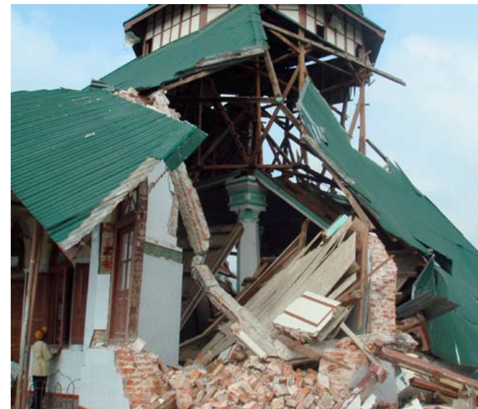
Figure 12. Collapse of a mosque is shown in these photographs. The URM walls on the extreme edges of the building collapsed due to the torsional motion.
