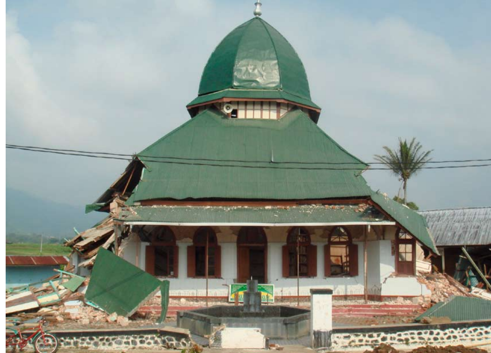
Figure 12. Collapse of a mosque is shown in these photographs. The URM walls on the extreme edges of the building collapsed due to the torsional motion.
