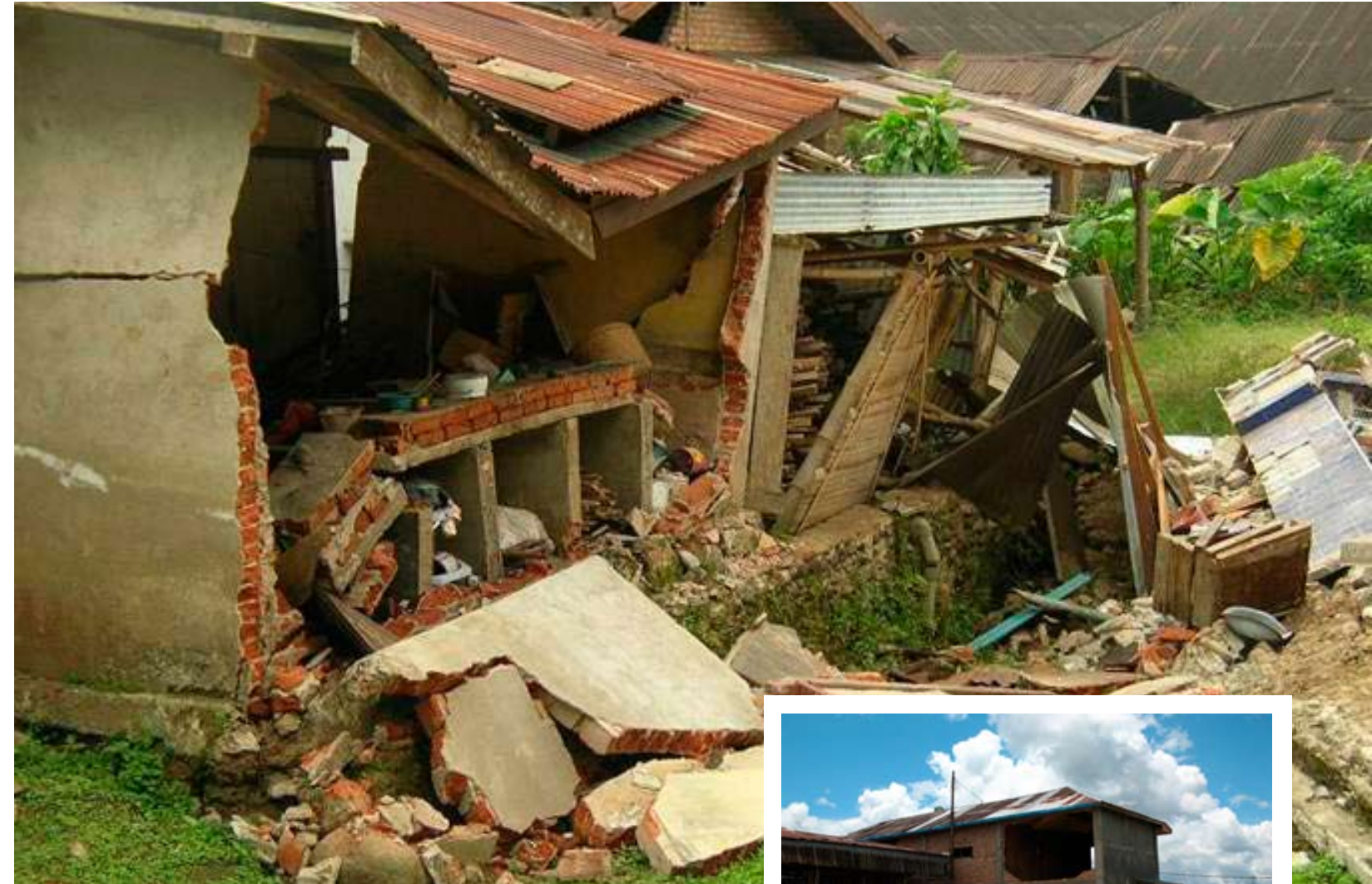
Figure 8. These photographs show out-of-plane failure of URM walls. These URM buildings do not have adequate floor diaphragms, and URM walls are not positively connected to the perimeter bond beams and columns. As such, they are not restrained against out-of-plane failure.
