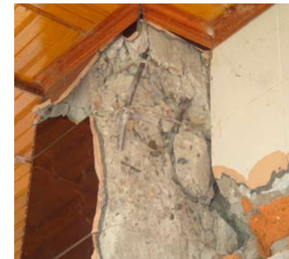
Figure 9. The beam-to-column joints for the concrete moment frames do not use ductile detailing. The reinforcement steel does not extend sufficiently into the joint, nor does it have adequate development length. Furthermore, the joints are not confined and hence are susceptible to shear failure.
