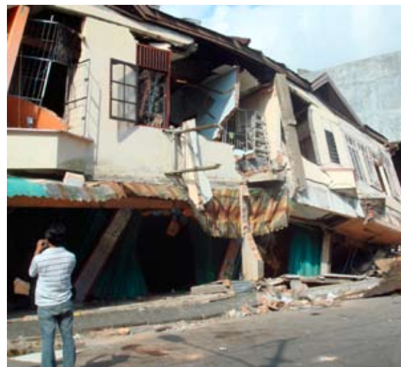
Figure 6. This commercial/residential structure used URM framing. The lateral-story stiffness and strength were significantly less for the upper floors and resulted in a soft-story collapse of the first story.
