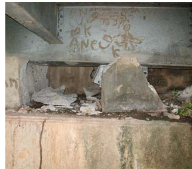
Figure 18. The photographs show failure of the substructure elements for the same steel truss bridge. The bridge is supported on bearings at the abutments, and it did not have an adequate transverse shear key. During the earthquake, the bridge slid off its bearings. The bearing pads did not have adequate width and/or restraint to allow or resist the seismic movement.
