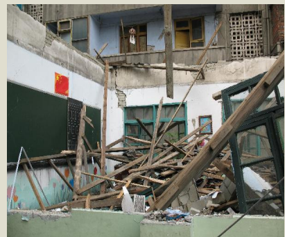
Piles of debris sit where Juyuan Middle School once stood.
