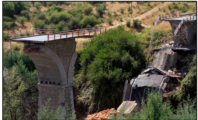
Upper right: USGS ShakeMap of the M8.8 earthquake, map of the area. Middle right: Older unreinforced masonry bridge over Claro river near Camarico, Chile. Lower left: A destroyed highway in Santiago, Chile, 200 miles from the epicenter. Lower right: A collapsed building in Concepcion, Chile located 70 miles from the epicenter.
