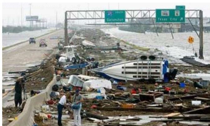
FIGURE 10. Roads were impassable in Galveston for many days following Hurricane Ike.
