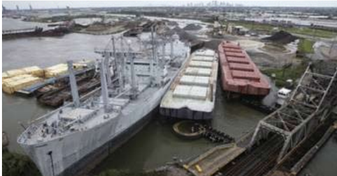
FIGURE 7. Numerous ships and barges broke their mooring lines and damaged each other, bridge supports, seawalls and docks, and blocked access to the industrial canal near New Orleans.
